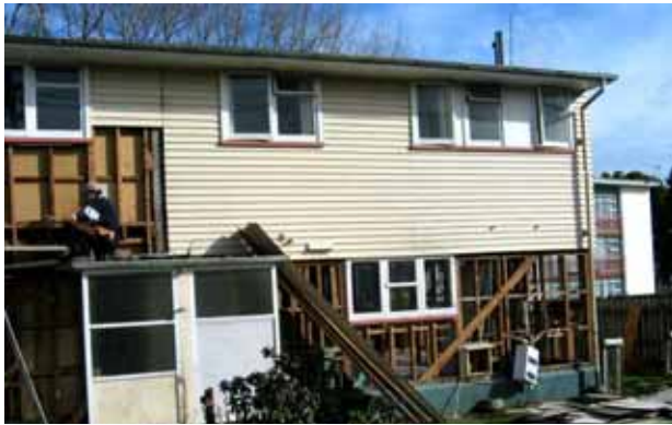
Salvage work on 1 st house commences prior to removal – August 2004
