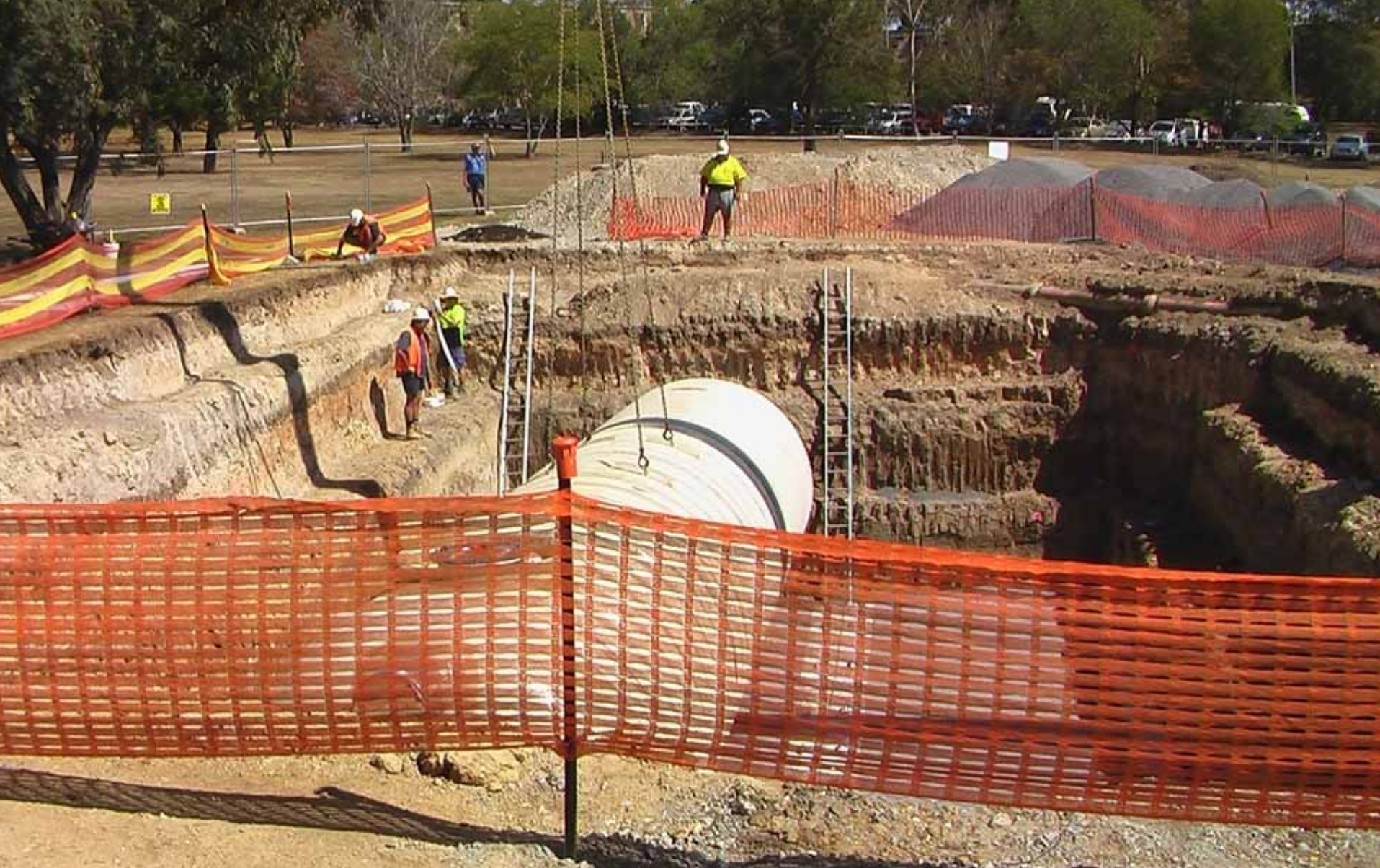
110,000 litre water tanks being installed at the University of Queensland
