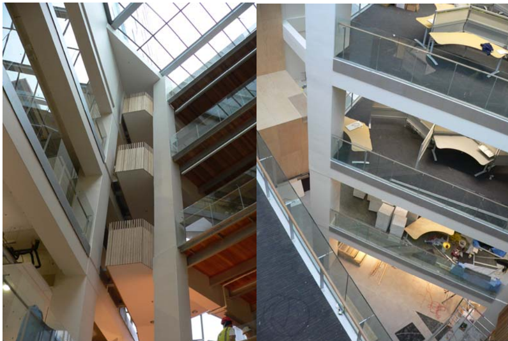
view of stairs with glazed atrium roof above
